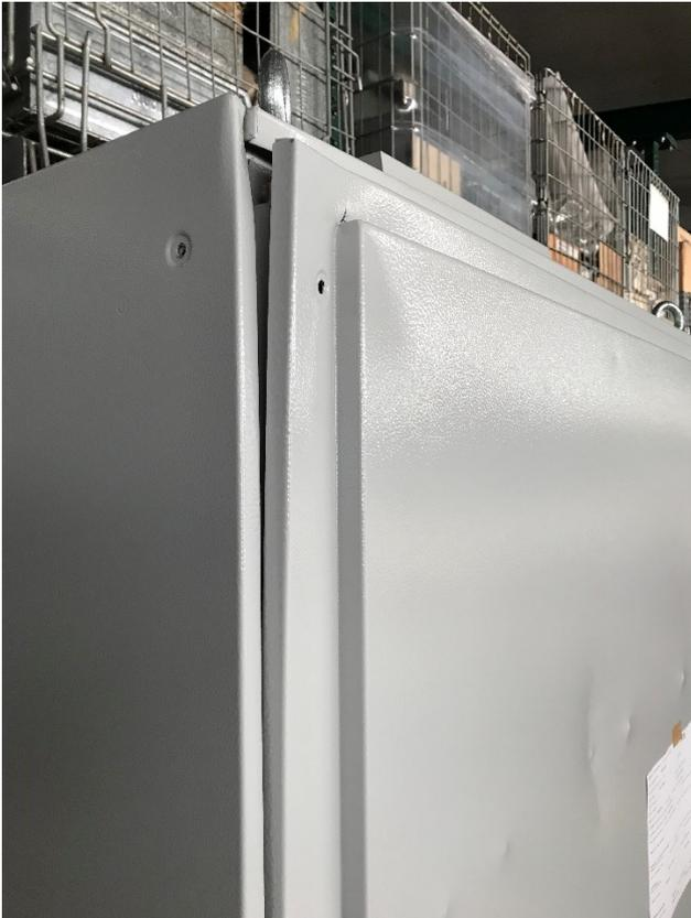
Outside panels of the AVR are damaged and have to be replaced:
